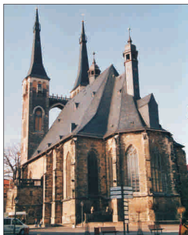
Cathedral of St. Jakob, 15th century, the oldest preserved building structure in Köthen
